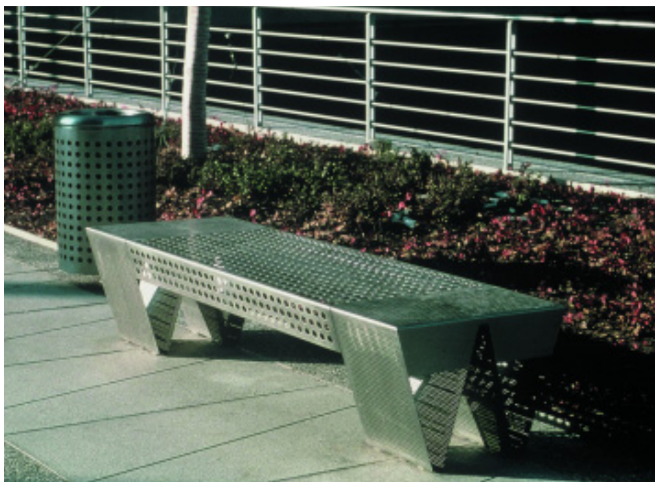
Figure A Specification of Type 316 stainless steel, a smooth finish and a design that takes advantage of rain washing keep this bench and handrail beautiful. (Photo credit – Paul Pittsford)
