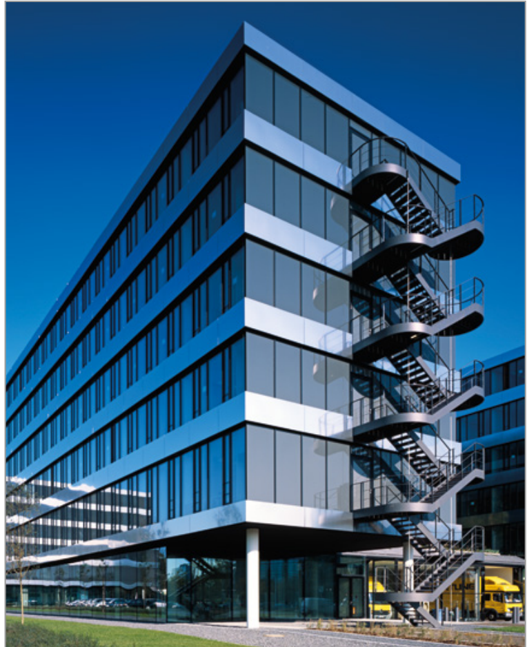
Adhesive bonding has been successfully used for stainless steel cladding for the façade. Photo: Ebener, Bad Marienberg (D)
