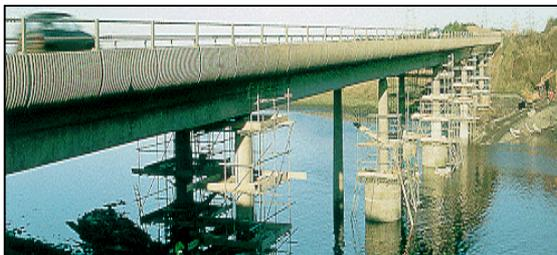
Figure 2 Example of concrete repairs to North Seaton Bridge
