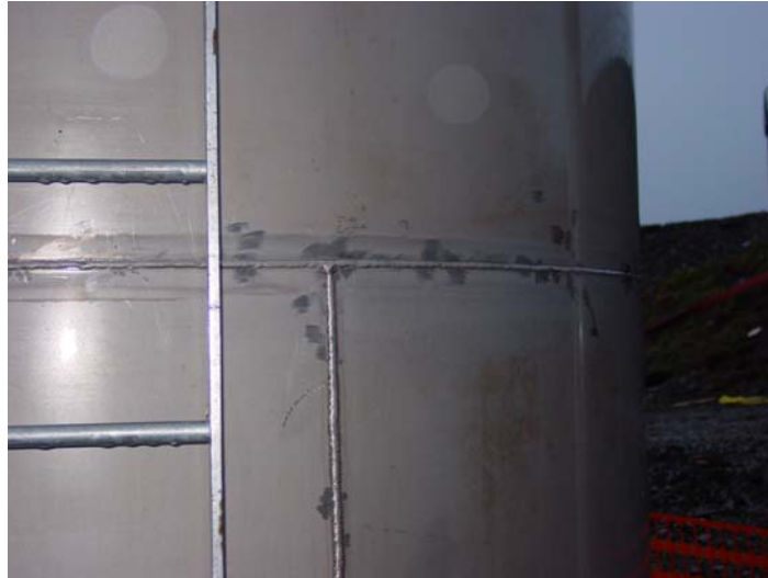
Fig 5. Welds on a tank after mechanical dressing and cleaning.
