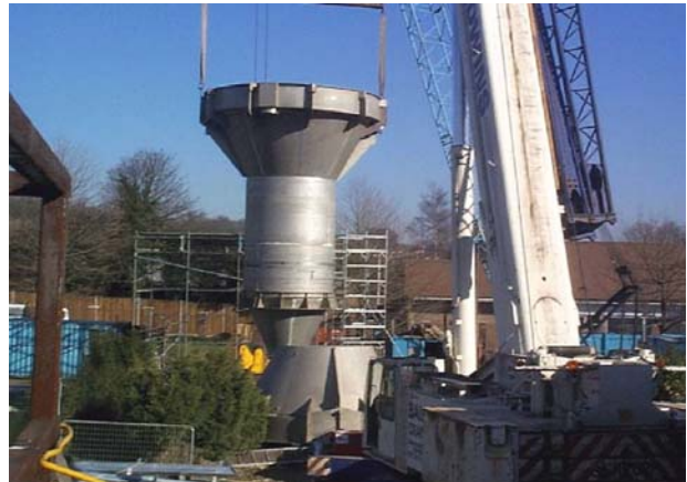
Installation of complete water softening reactor
